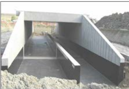
Completed Structure in July 2010
