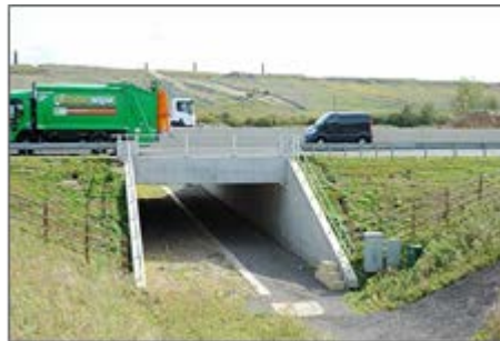
Completed road open for traffic
