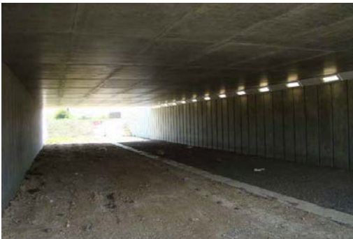
Tunnel showing lighting
